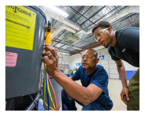
HVACR technicians install, maintain, and repair heating, cooling, and refrigeration systems.
